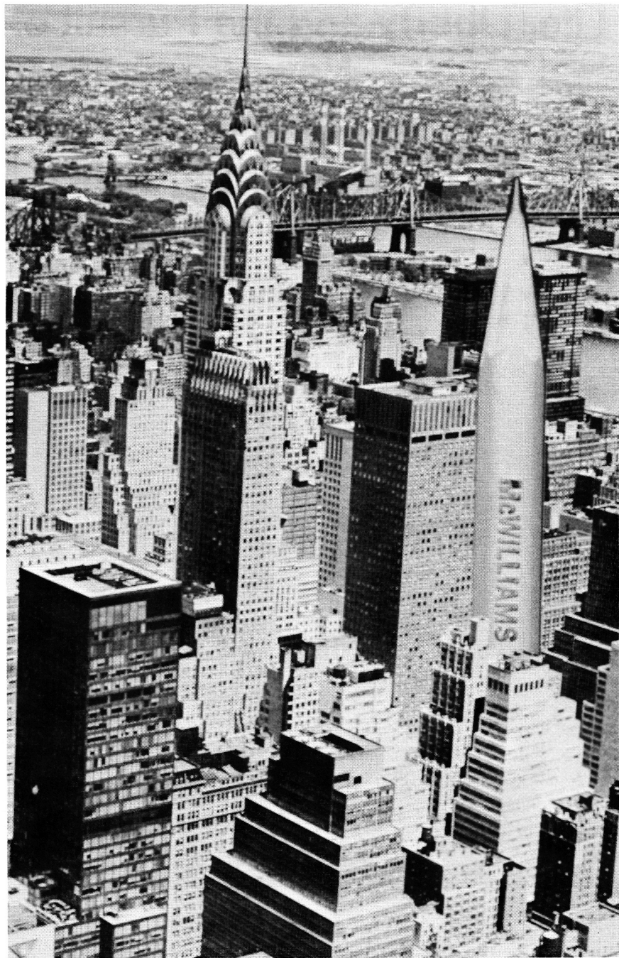
The McWilliams Building.
